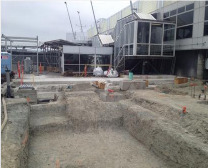
C2 – Elevator Pit and Stem Wall Excavations
