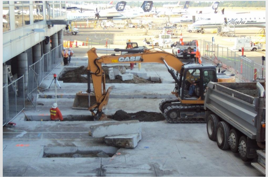
C16 – Grade Beam Excavations and Panel Removals
