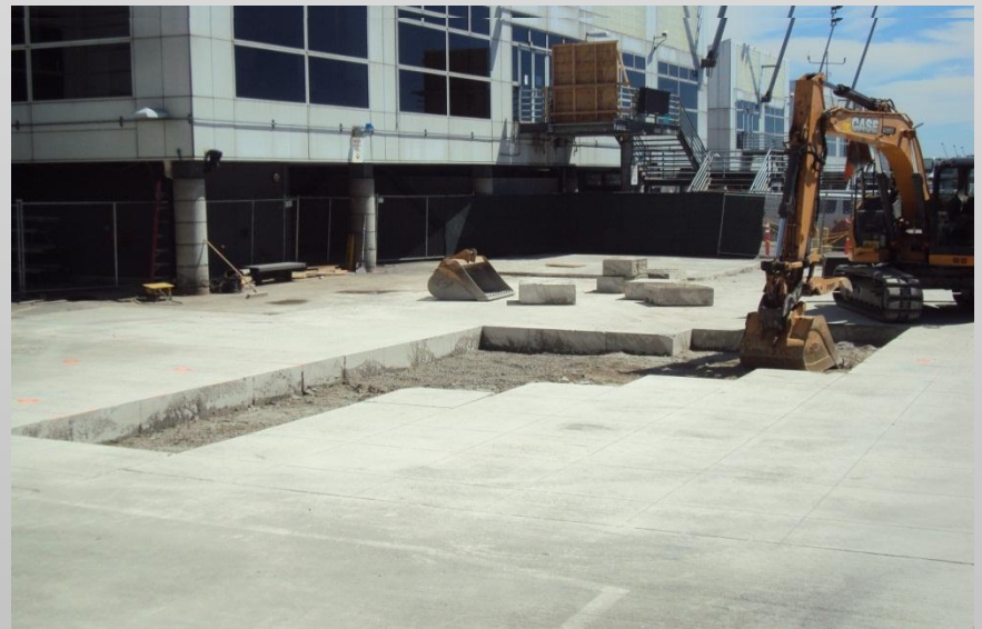
C10 - Removal of Pavement for Waterline Relocation
