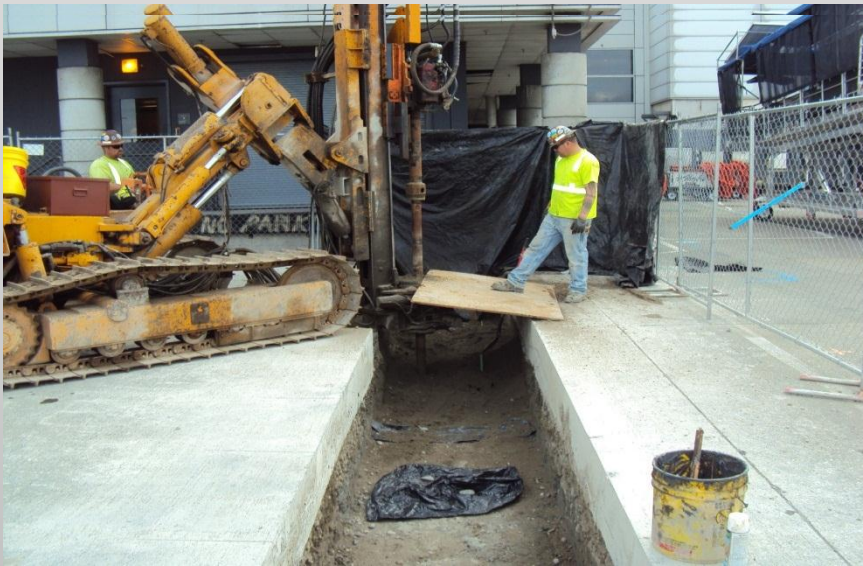
C2 – Micropile Installation
